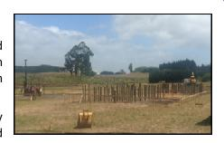
The first order of business for the contractors were the trenches for the common services and preparing the sites for the piles of the whare. The contractors then started laying the floors, followed by the erection of the prefabricated framework for the 5 whare. All of the rooftops are now on and the aluminium joinery has been fitted into place, currently the builders are working on lining the exterior and interior of the whare.
